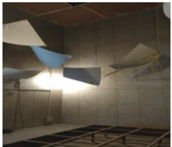
Anechoic chamber and Reverberation Chamber at CSIR-NPL for Acoustic Characterizations
