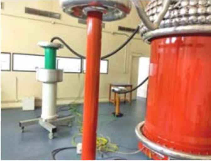
Calibration set-up for 200kV AC High Voltage Divider
