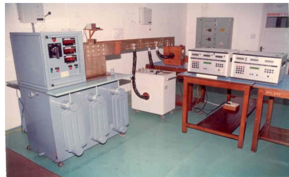
AC High Current Setup upto 5kA made for 200kV Divider
